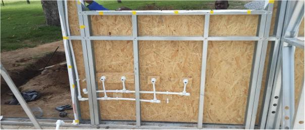
All electrical and water reticulation is installed within the light weight frame walls,
